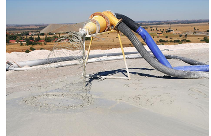
(c) Cyclone Deposition (preferred)
